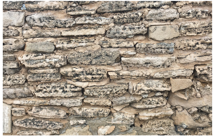
An example of the Calcarenite as found in Slaughter Bay. Note sound condition given the exposed location. Source: Purcell.
